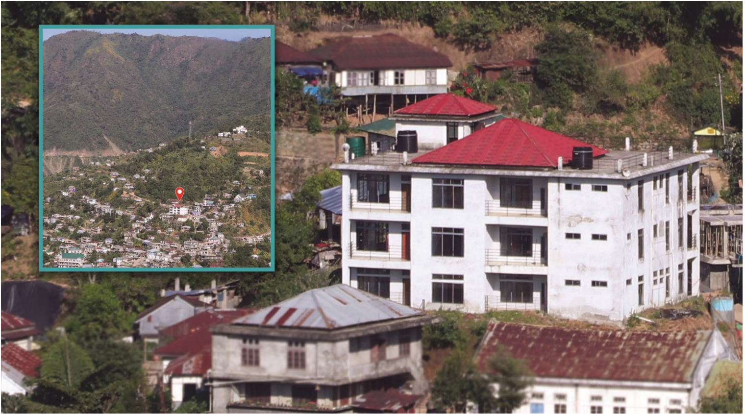
The building in focus is the Hostel of Member of District Council (MDC), MADC at Siahatláh, Siaha
